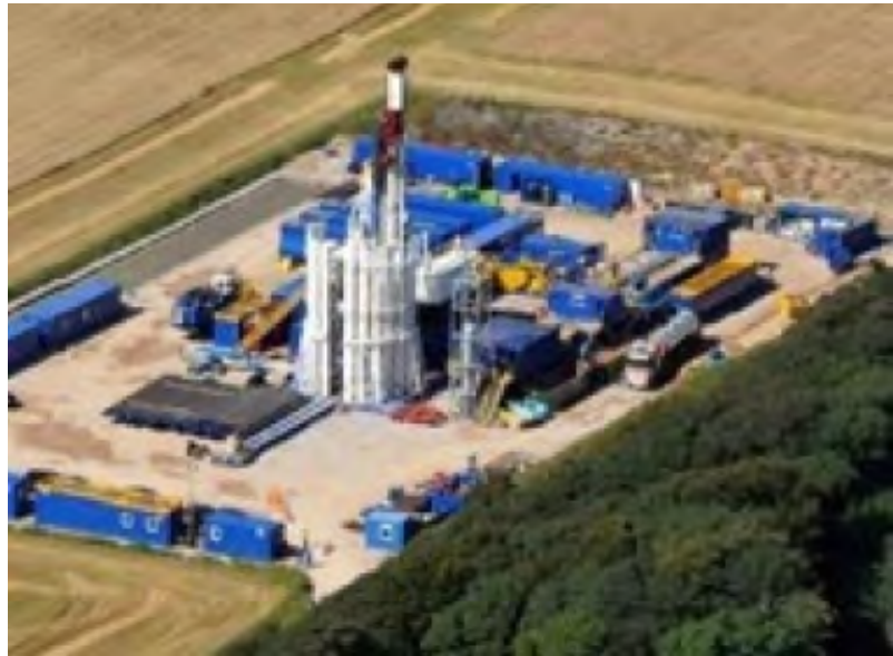
Shale gas extraction rig Photo c Brian Jones
