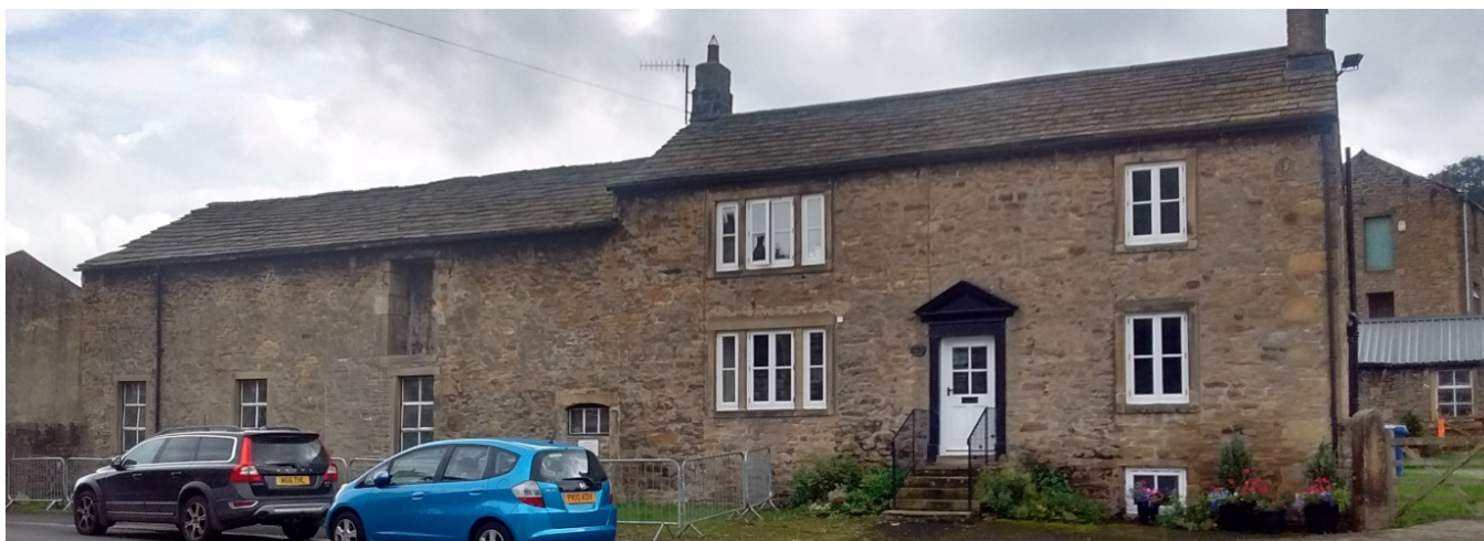
Fig 19 Grundy Farm with listed wall attached; largely unaltered since the nineteenth century
