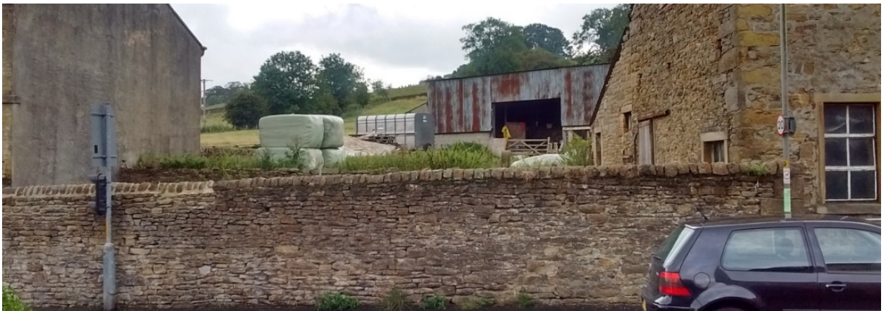
Fig 10 View directly towards listed wall and into application site from 1 & 2 South View
