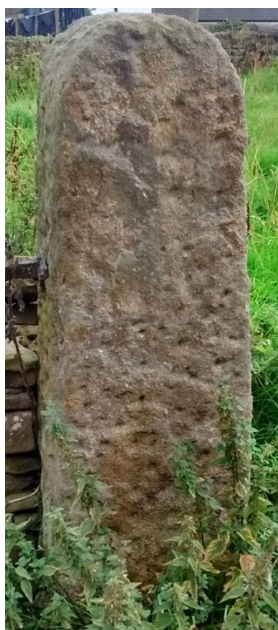
Fig 5 Monolithic gatepost forming part of enclosure to be demolished
